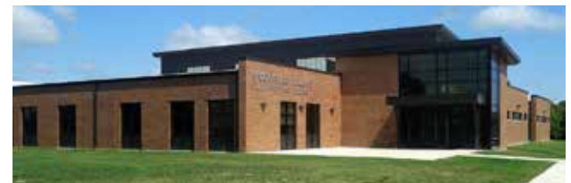
Visit our newly constructed Multi-Purpose Building
