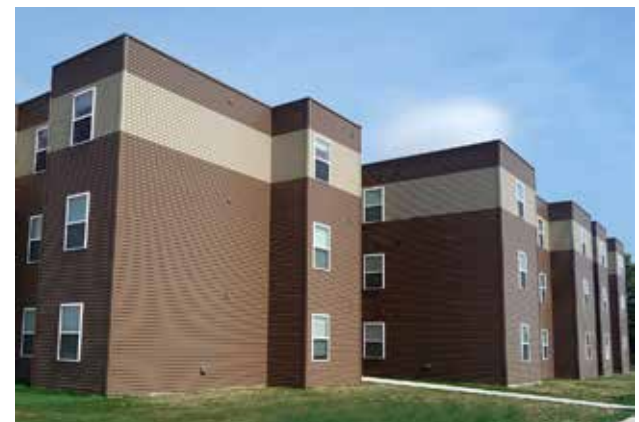
Tour the Snapper Villas (on-campus housing)
